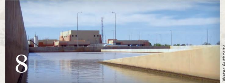
After being diverted, the water is pumped uphill from the Rio Grande for storage and treatment at a **surface-water treatment plant** (8) on Albuquerque's north side. From the plant, the water can be distributed throughout the utility's service area in Albuquerque and Bernalillo County.
