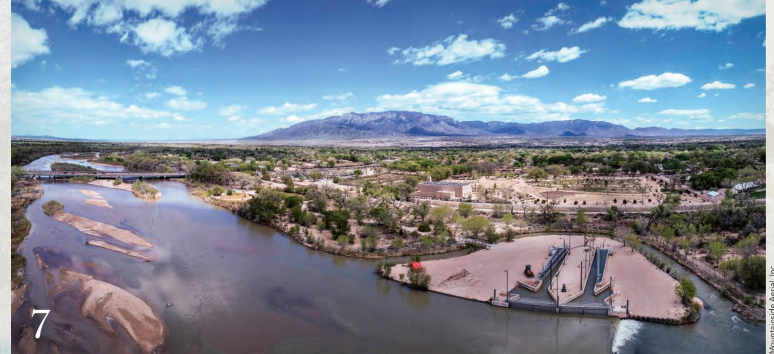
After traveling about 150 miles from Colorado, San Juan-Chama water eventually arrives in Albuquerque. An **intake facility** (7), including an adjustable dam and fish passage, diverts the water to the pump station for processing.
