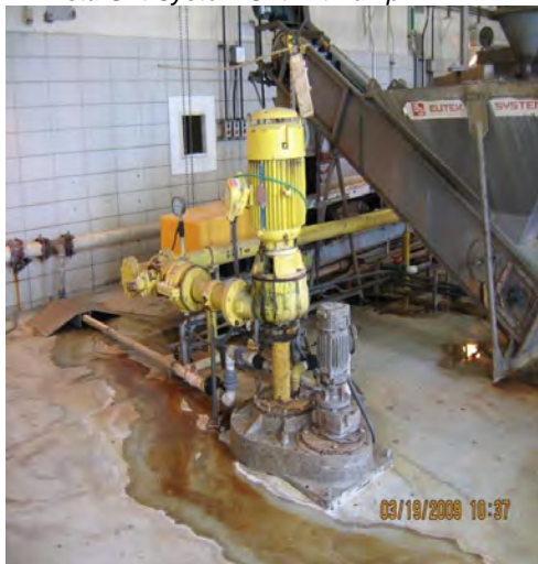
PTF Pista Grit System Grit Lift Pump
