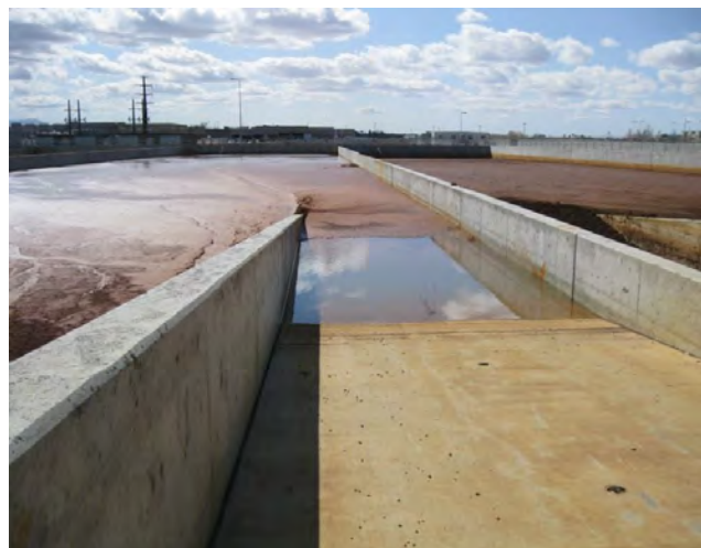
Ramp of Sludge Drying Bed at SJCWTP
