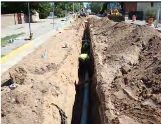
New 6-inch Water Line Installation
