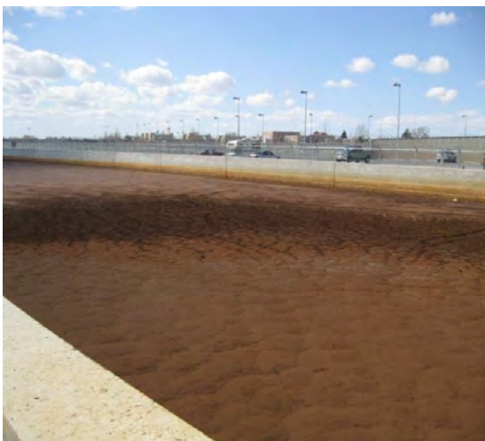
Sludge Drying Bed at SJCWTP
