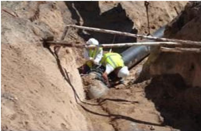
**24” Concrete Cylinder Water Line Lowering and Relocation for a City Storm Drain Project in San Mateo NE**
