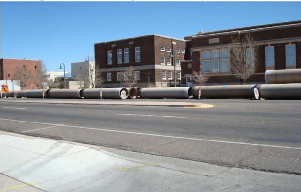
**New 27-inch Sewer Line Sliplined in the old 30” Concrete Pipe in Prospect NE west of Carlisle**
