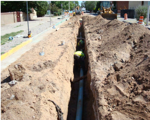
New 6-inch Water Line Installation
