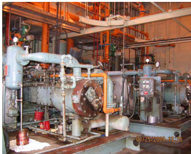
Gas Compression Compressors to be replaced
