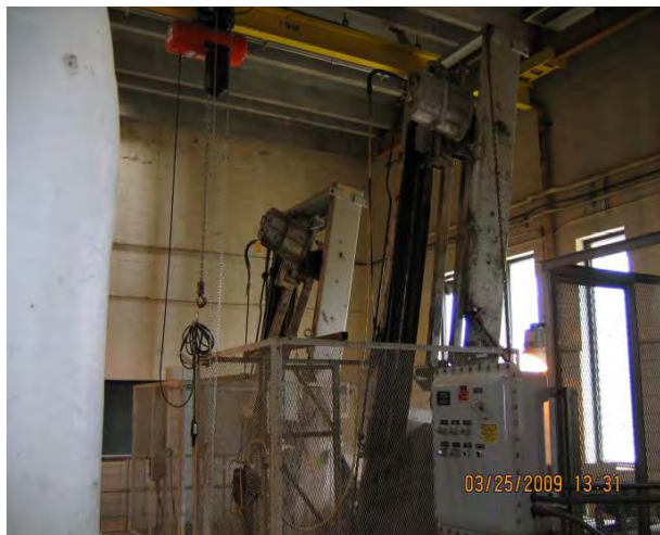
PTF Lower Barscreens to be replaced
