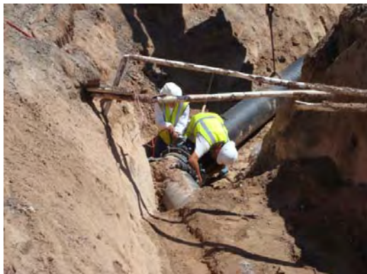
16" Ductile Iron Water Line Relocation for a City Storm Drain Project in Atrisco SW
