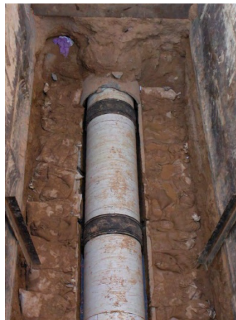
New 27-inch Sewer Line Slip-lined in the old 30" Concrete Pipe in Prospect NE west of Carlisle
