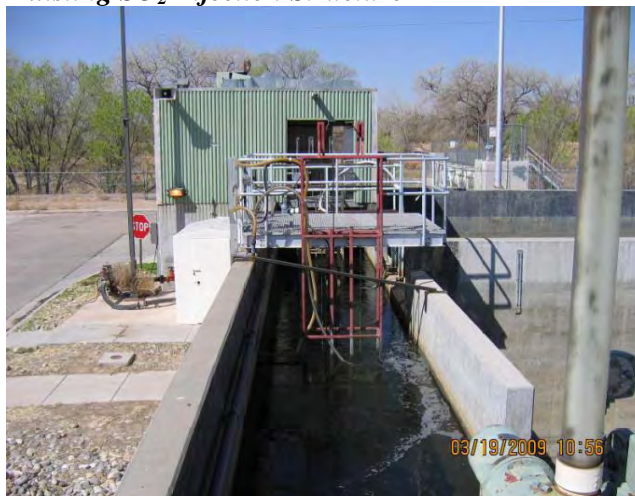
Existing SO 2 Injection Structure
