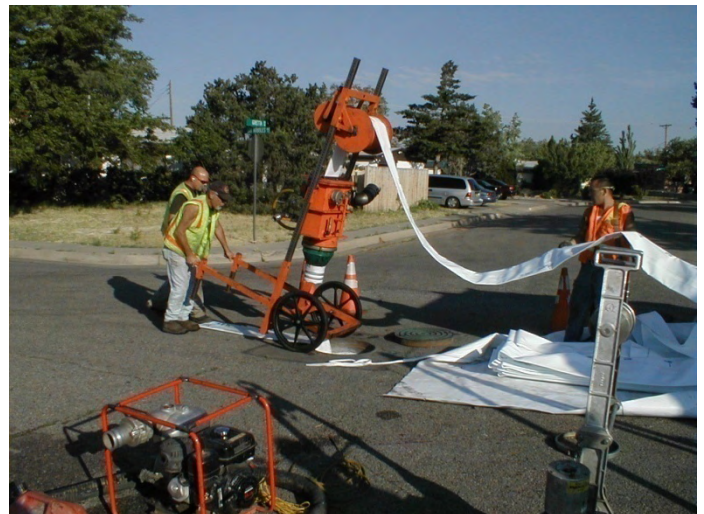
8-inch Sewer Lining Project on Los Arboles NE
