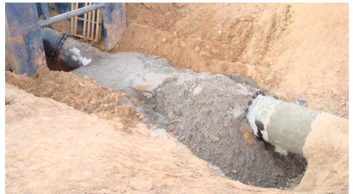
24" Concrete Cylinder Water Line Lowering and Relocation for a City Storm Drain Project in San Mateo NE
