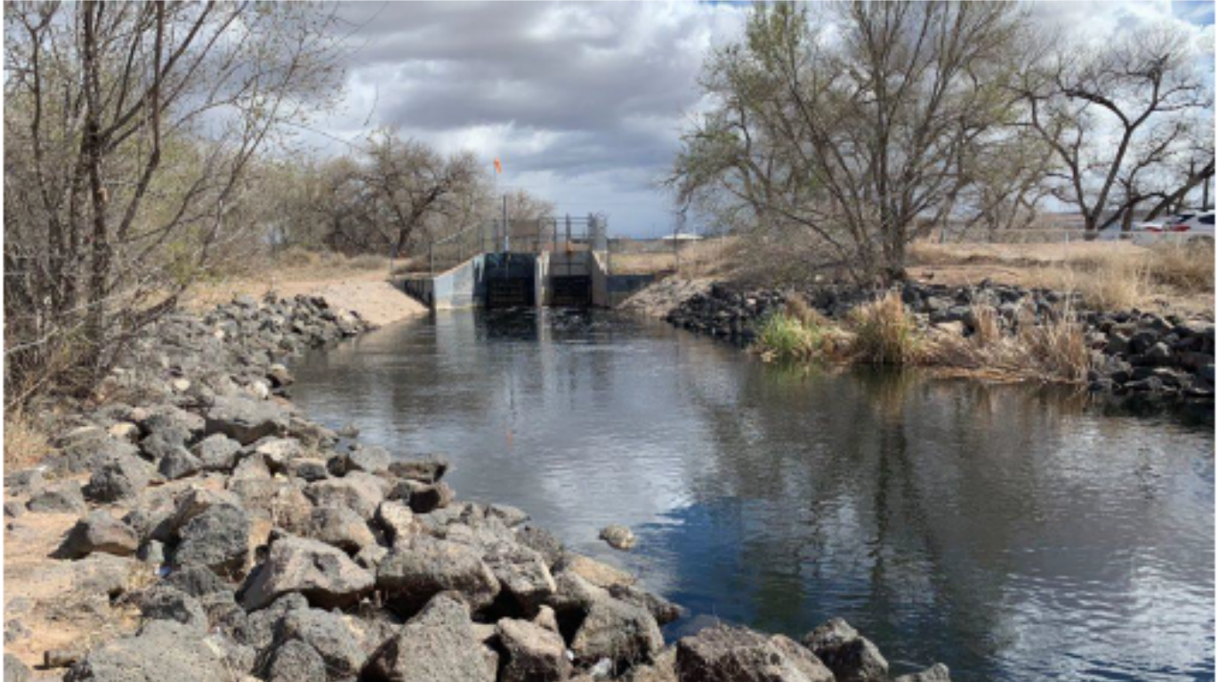
Southside Water Reclamation Plant Outfall Structure
