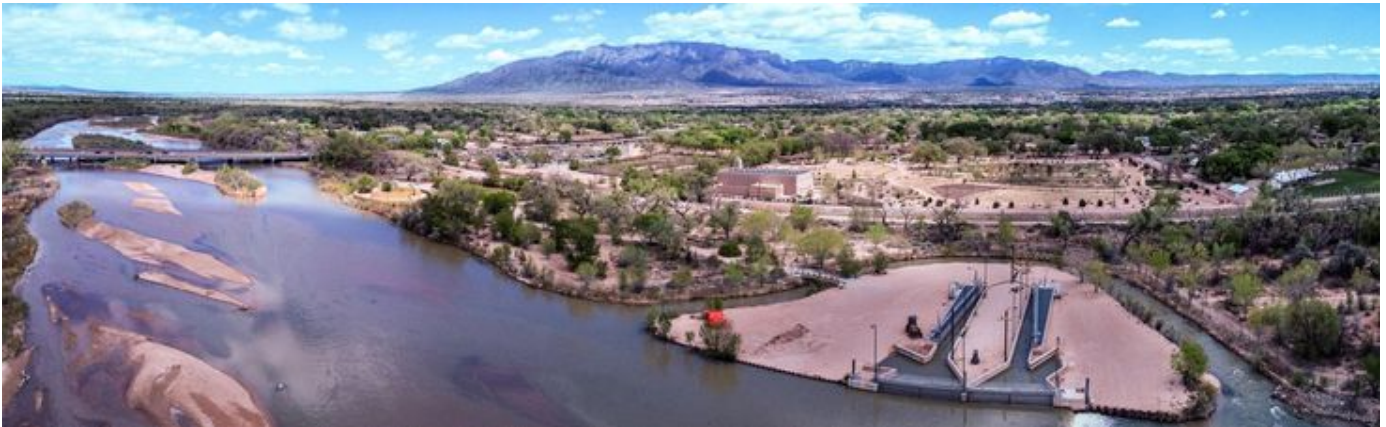
San Juan-Chama Diversion Dam
