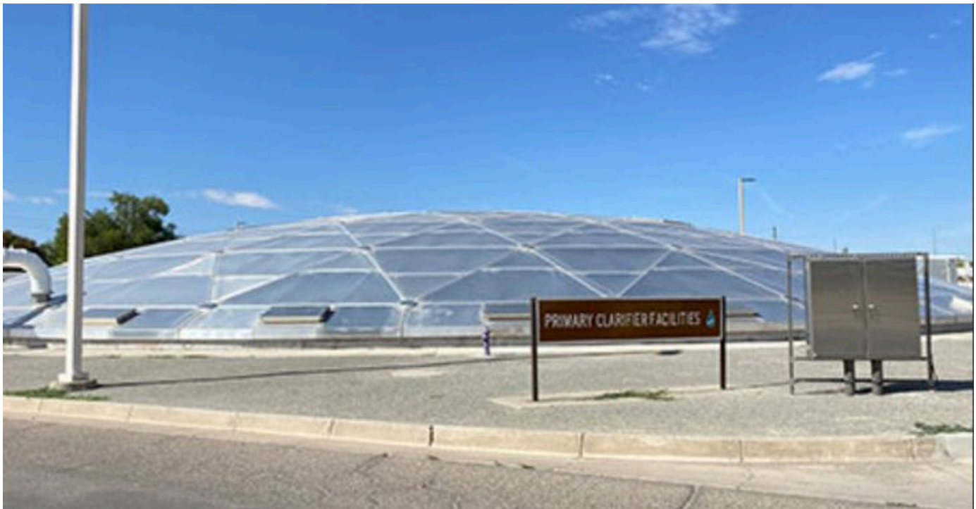
Southside Water Reclamation Plant Primary Clarifier
