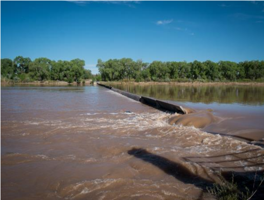
Diversion Dam off the Rio Grande River
