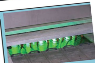
Disinfection Ultraviolet light destroys genetic material in bacteria and viruses.
