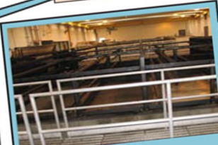
Thickening Sludge is thickened and de-watered before it goes to the digester.
