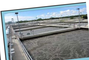
Aeration Basin Bacteria eat the dissolved solids and denitrify ammonia into nitrogen gas.
