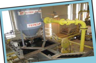
Grit Chamber Sand, grit, coffee grounds, and egg shells settle out here.
