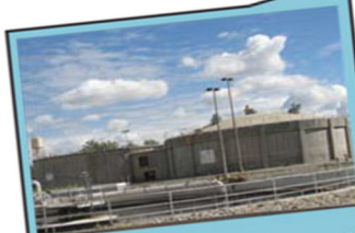
Digesters Microorganisms kept at 98 degrees F produce methane gas.
