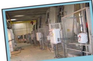
Bar Screens Giant rakes allow water to pass, but catch trash like sticks, rags, and toys.
