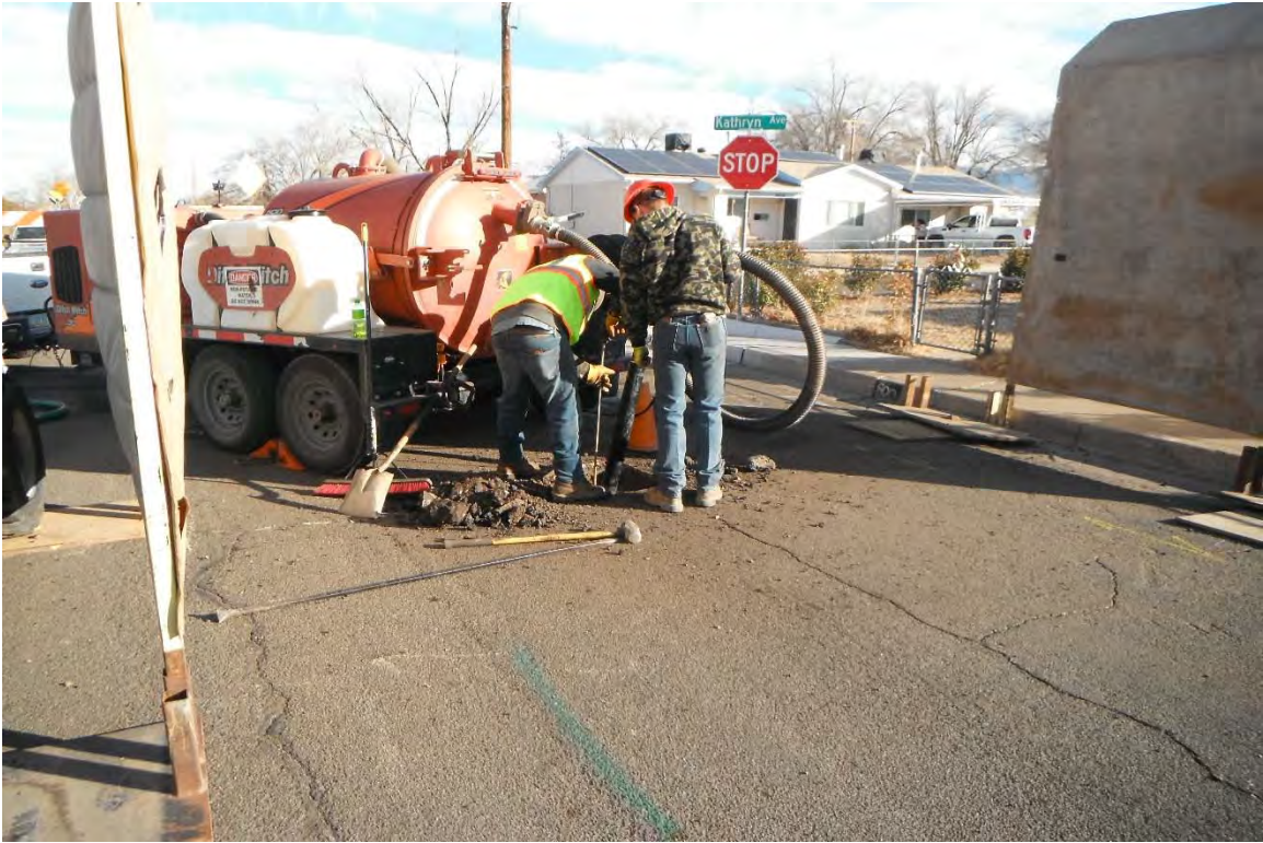
No. 3 – Daylighting activities and sound panel placement.
