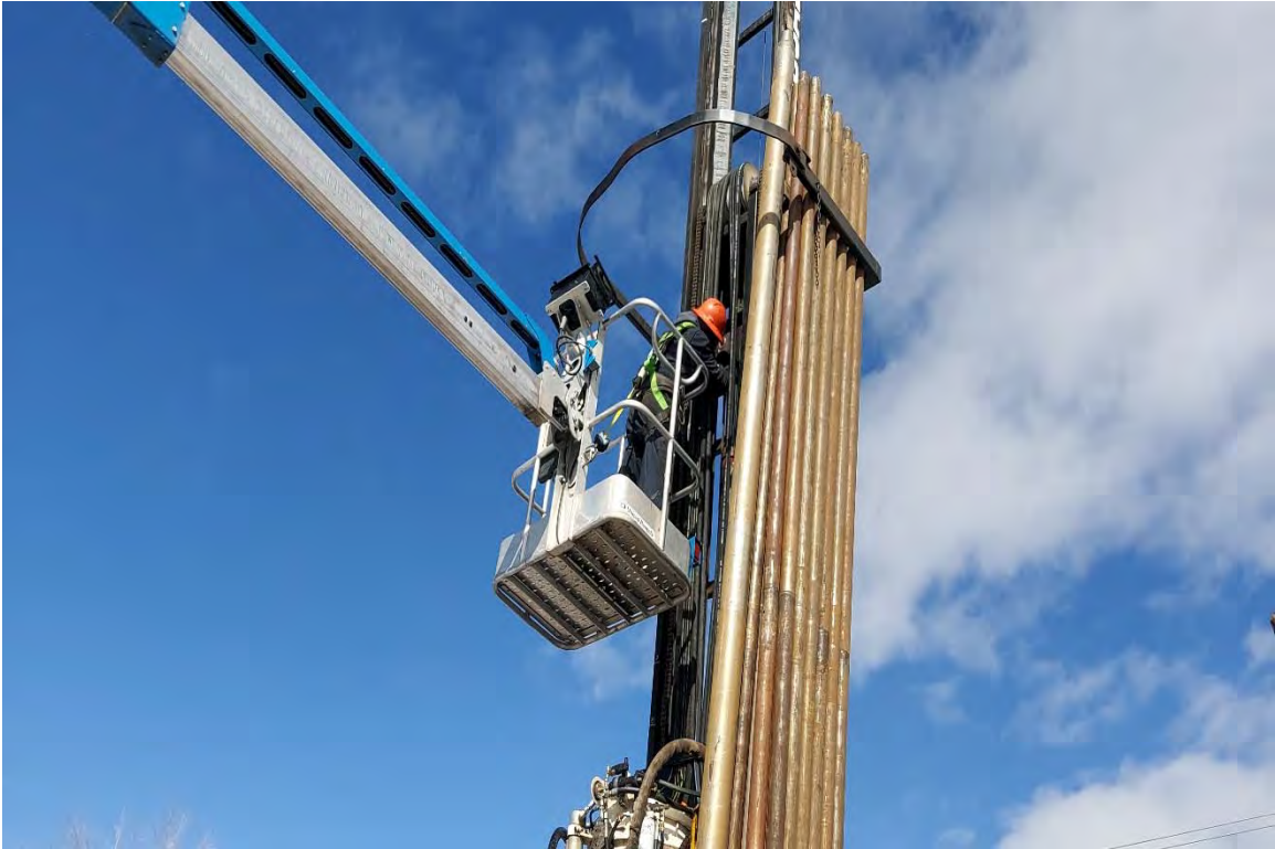
No. 16 – Rig Repair at mast using high-lift.
