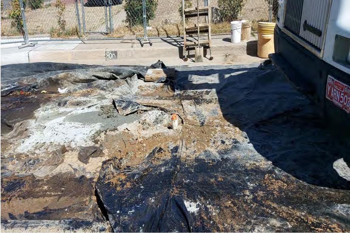
No. 23 – Monitoring well installation with locking cap.
