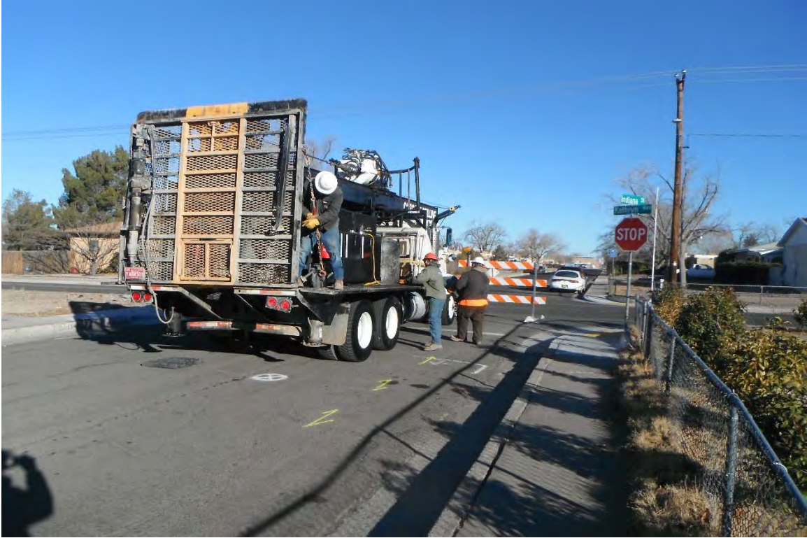
No. 1 – Confirming rig will meet layout requirements
