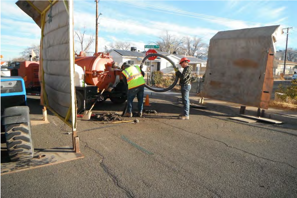
No. 2 – Daylighting activities and sound panel placement.
