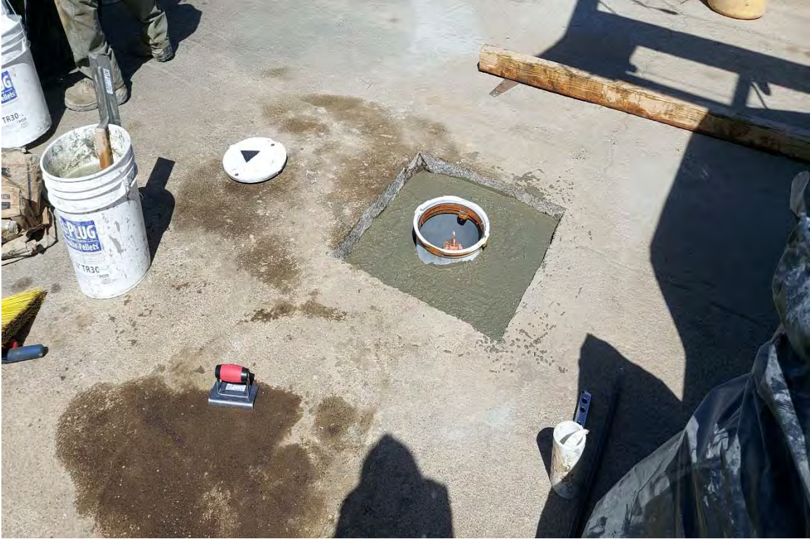
No. 25 – Concrete Pouring – monitoring wellhead post inspection approval.
