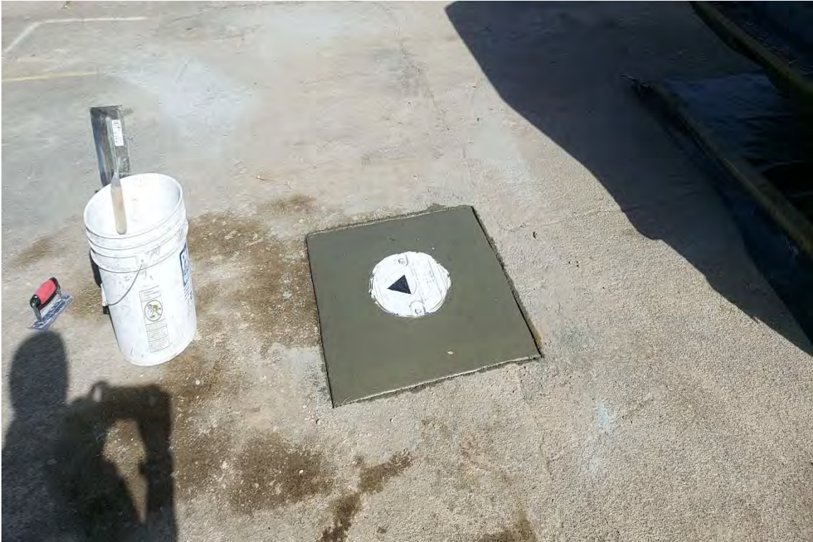
No. 26 – Final monitoring well installation – Data Gap Monitoring Well WUABFFMW01.
