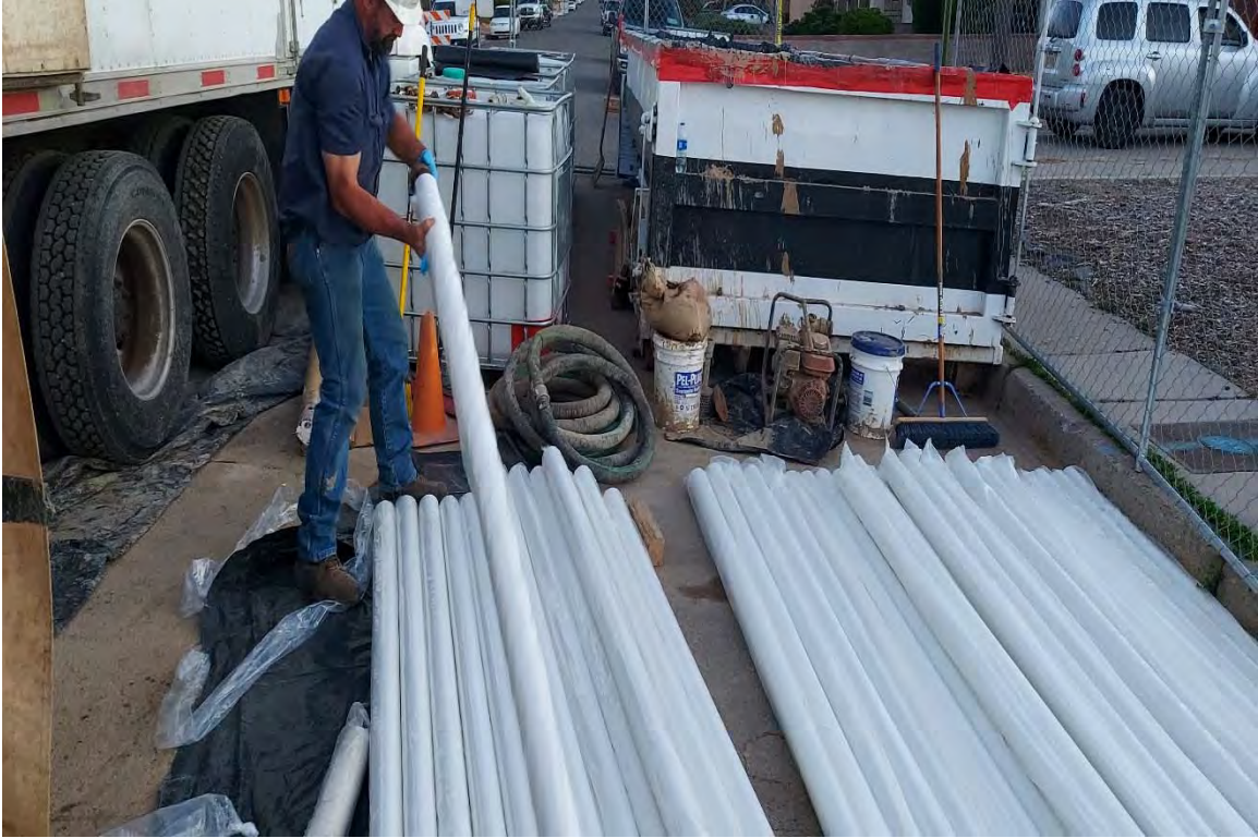
No. 19 – Preparing Well Casing for Monitoring Well Installation.
