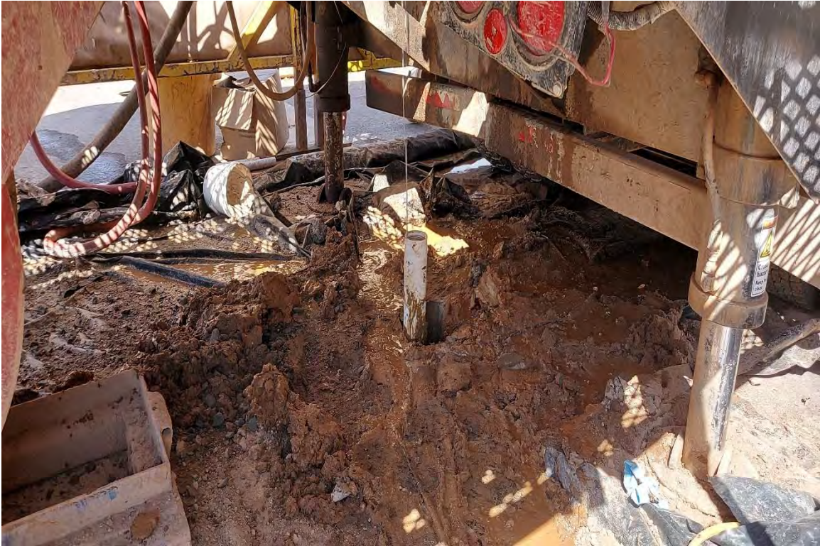
No. 22 – Monitoring Well installation – final section of monitoring well casing.
