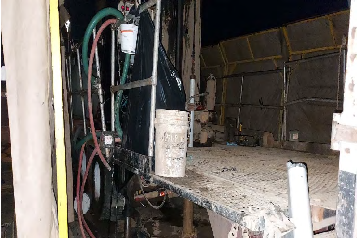
No. 20 – Monitoring Well casing installation.
