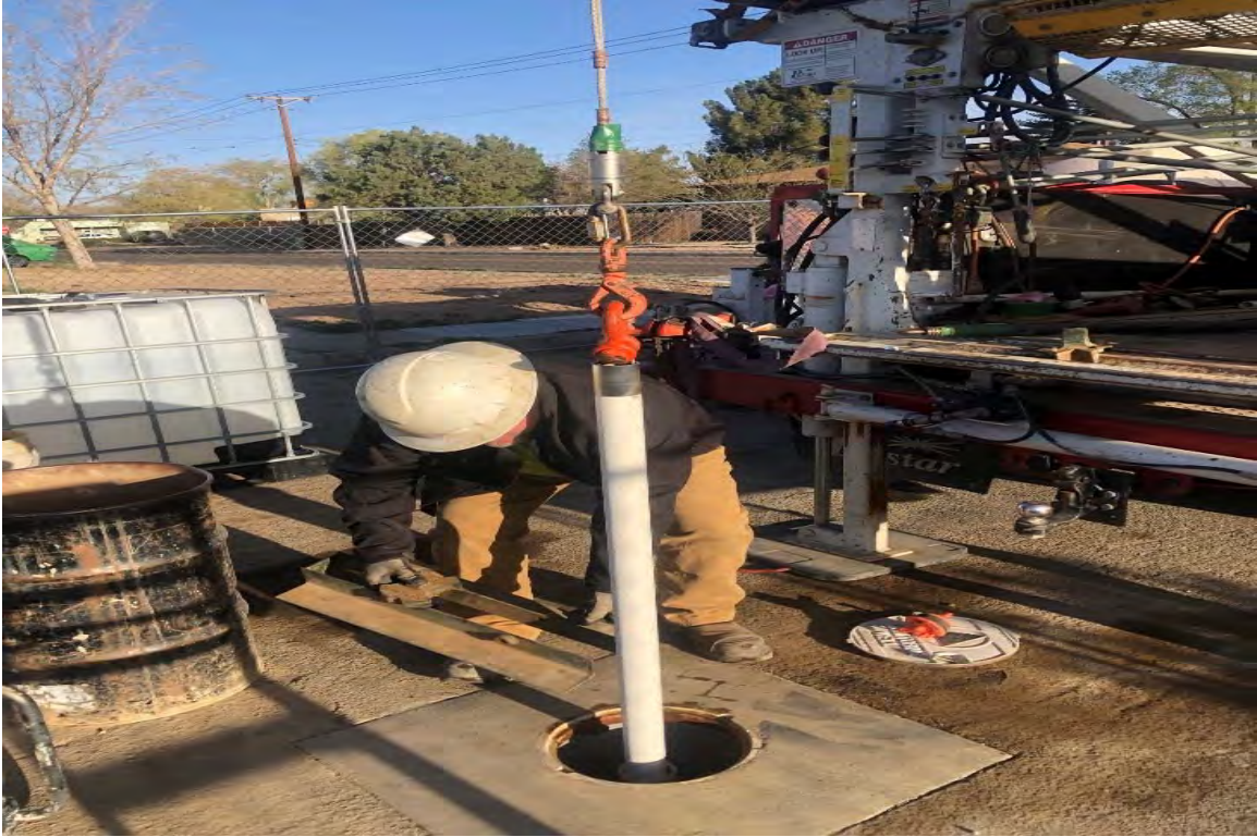
No. 27 – Photograph of WUABFFMW01 during development. The well was being bailed.
