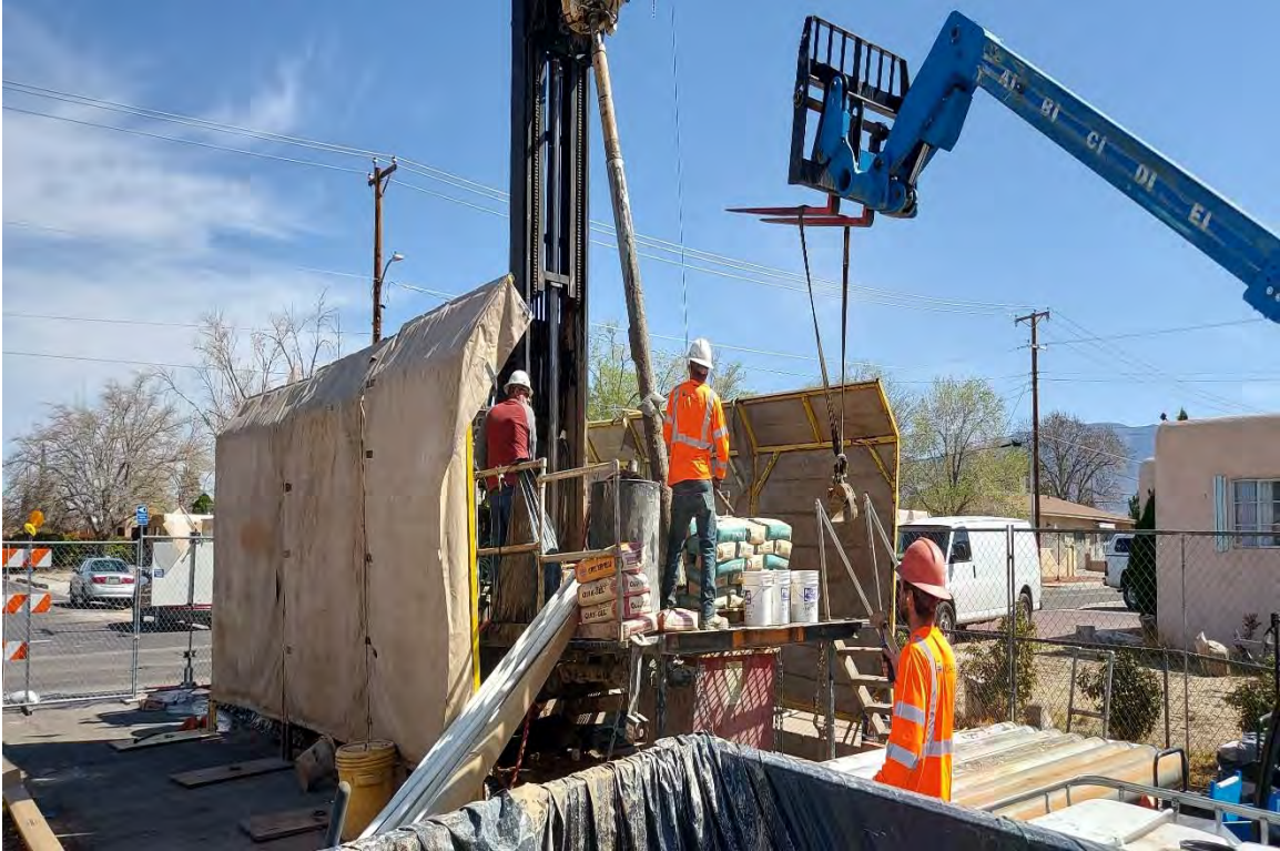
No. 21 – Well installation materials/removal of final section of drill casing.
