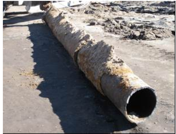
Corroded Steel Pipe
