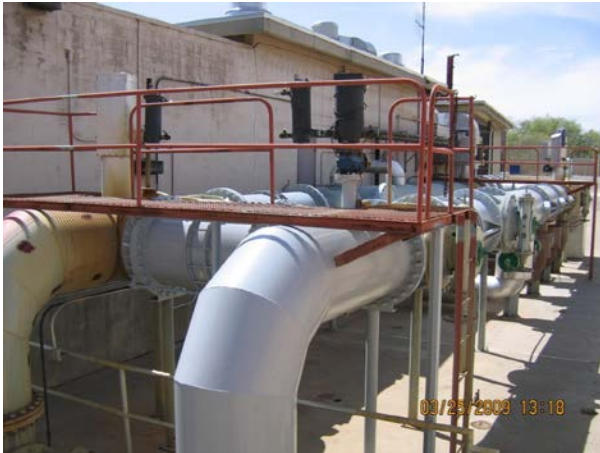
Lift Station #20 Force Main Header
