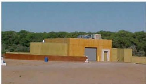
Nonpotable pump station located near the Rio Grande.
